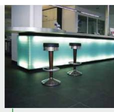
Fibreglass is versatile for example, counters and other structures can be cladded with it.
